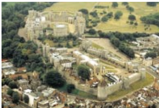
Windsor Castle showing, bottom left, St. George's House and Chapel.
